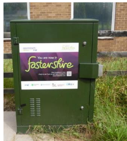
Fibre Enabled Fastershire / Openreach Cabinet
