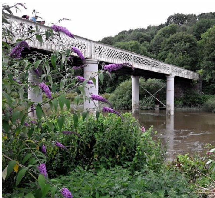
Brockweir Bridge, River Wye, Western Border Hewelsfield and Brockweir Parish
